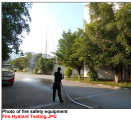
Photo of fire safety equipment Fire Hydrant Testing.JPG
