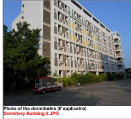
Photo of the dormitories (if applicable) Dormitory Building-2.JPG
